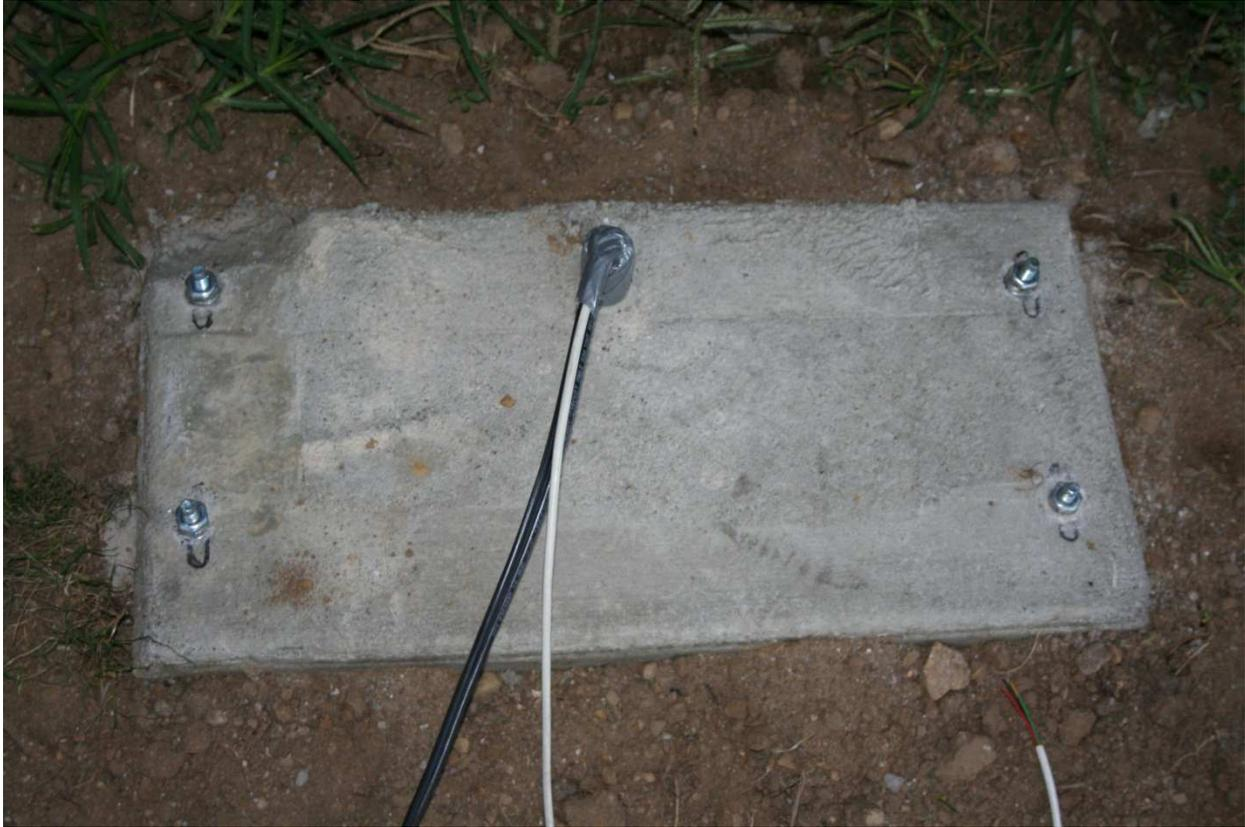
Here is the pad with the conduit trimmed to about 1 inch above the surface and the wiring wrapped in duct tape to try and keep the water out. The supplied anchor bolts have been installed.
