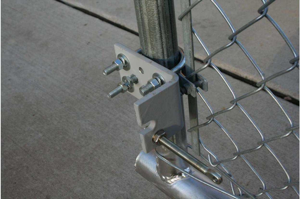
These are photos of the brackets in place on the gate. Some show the tension bolts attached. The belt mounts to the hole at the end of the bolts.
