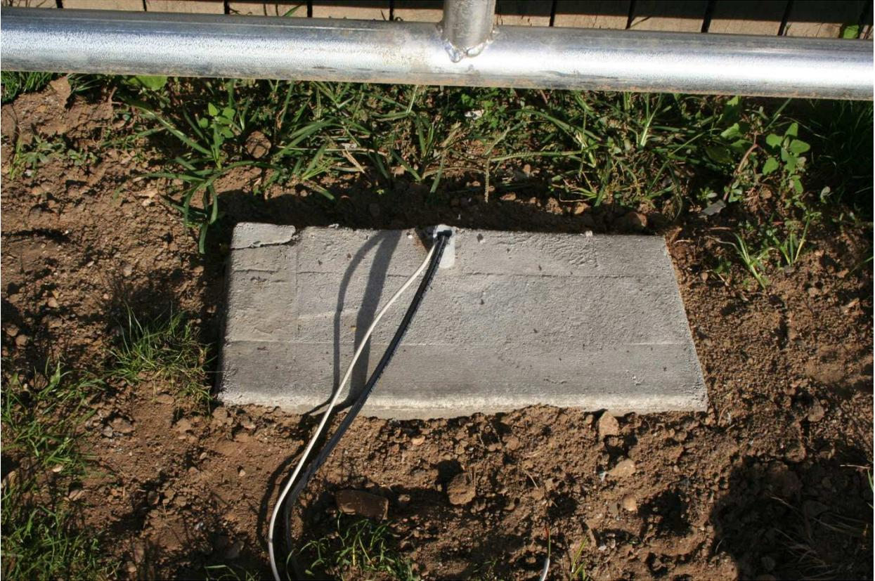
The pad once the concrete had dried and the form removed. Note the conduit and the power & phone wiring.
