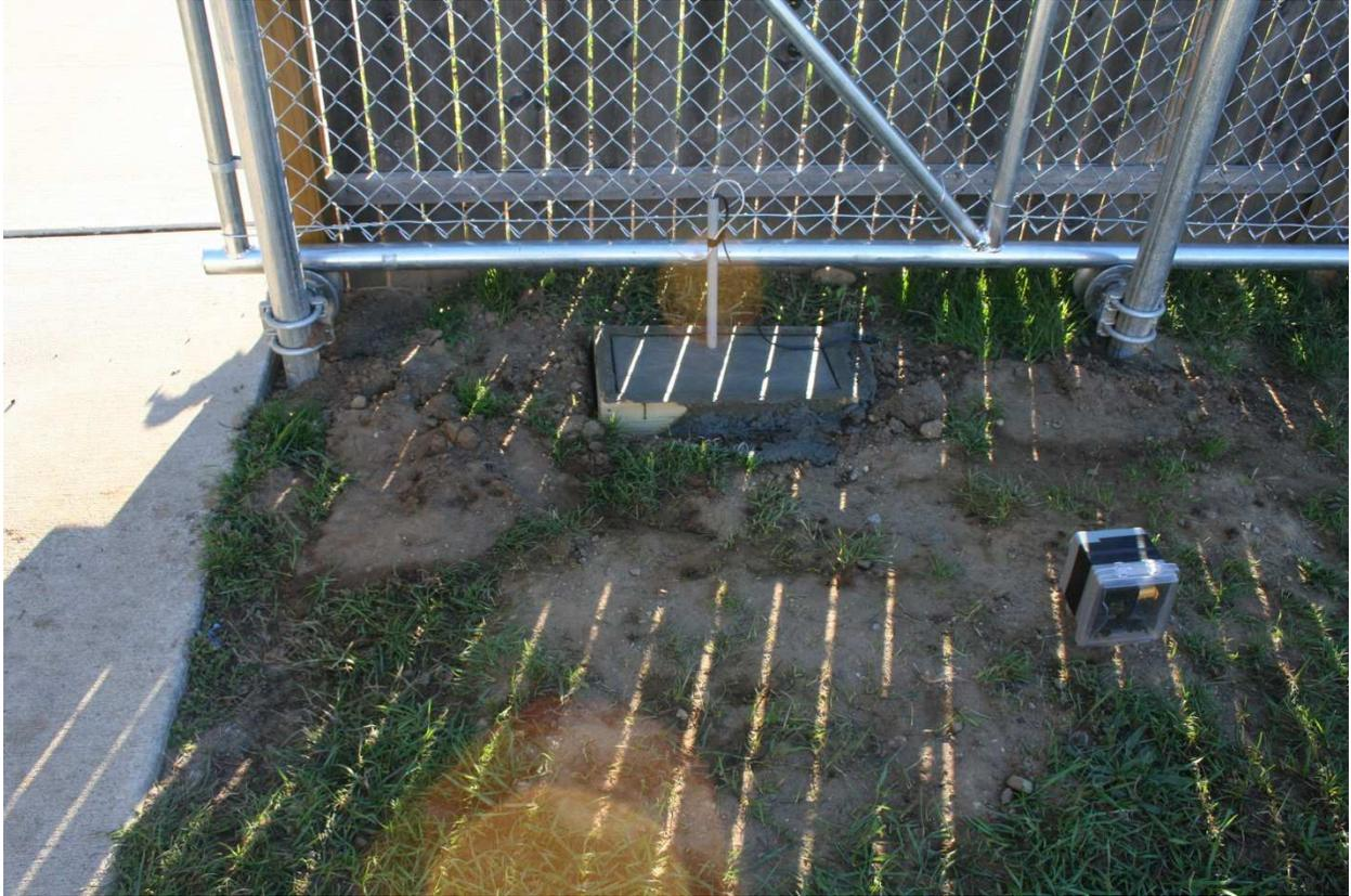
Fresh concrete in a wooden form is shown above. Please notice the outlet box. ½ inch PVC conduit is buried 18-in below ground between the two. If I were to do this again, I would have added about 2-3 inches to the height and width of the pad. The suggested size puts the concrete anchor bolts a little too close to the corners: the concrete split when I torqued the bolts into position. We patched it up and tried to waterproof the whole thing. See my UPDATE discussion later in this document.
