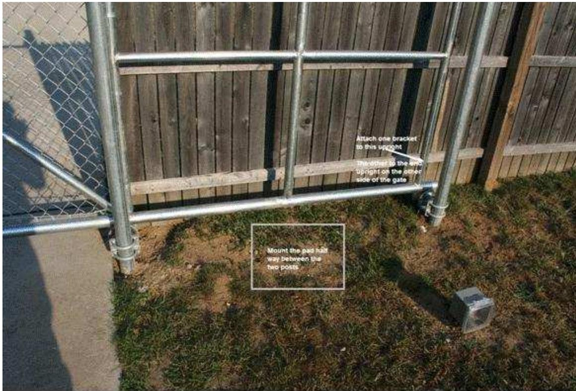
OK. So construction started. First order of business was to get power to the site. I was very fortunate in that I had already installed 120VAC to a free-standing outlet box close to the gate (you can see the original outlet box at the lower right of the above photo). I dug a short trench and put in some conduit between the outlet box and the pad site.
