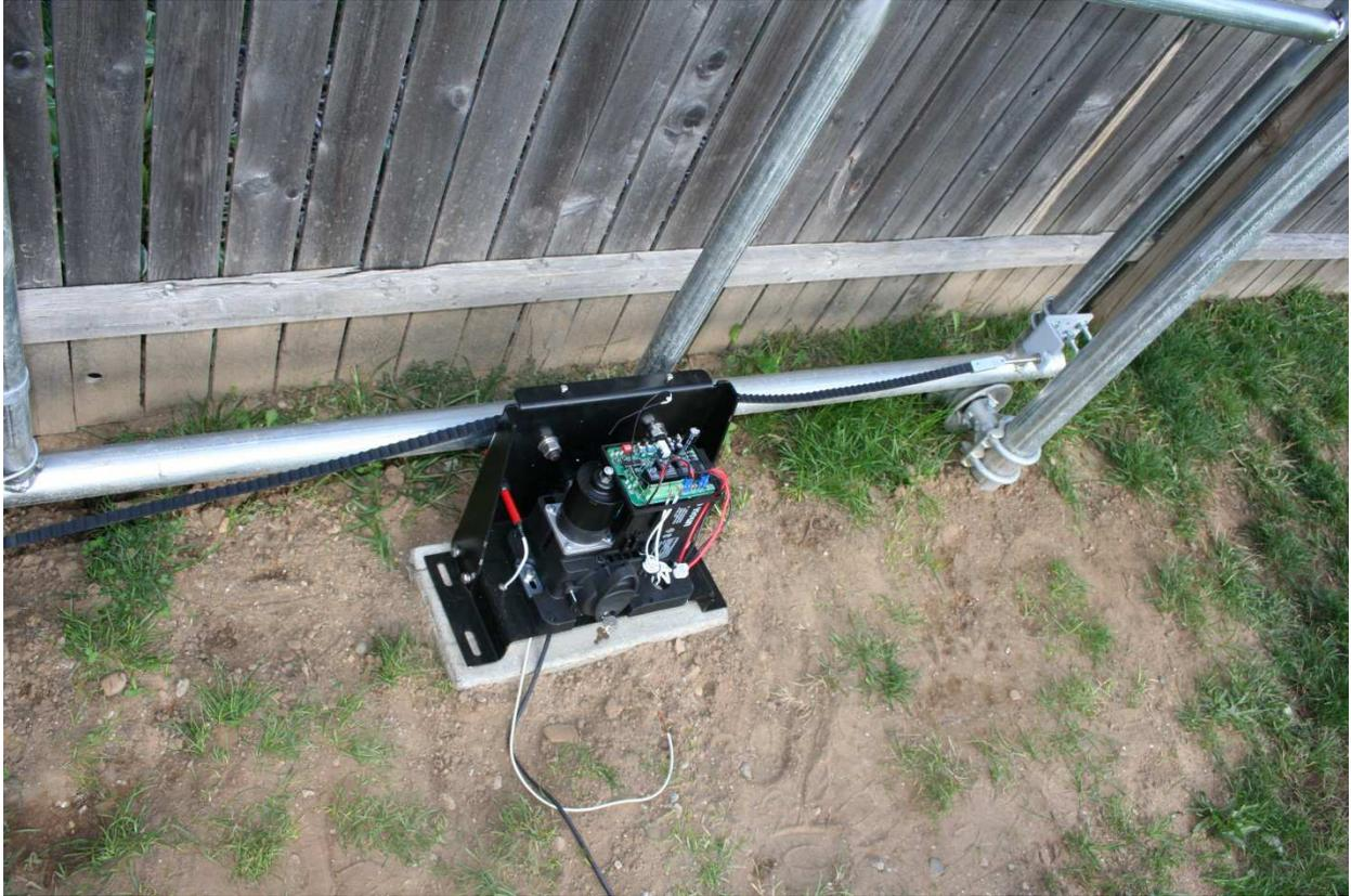
These are photos of my first dry fit. The belt is threaded through the opener and excess removed as described earlier. Once the base is bolted to the slab tighten the belt using the nuts on the tensioning bolts as shown in the next photo.
