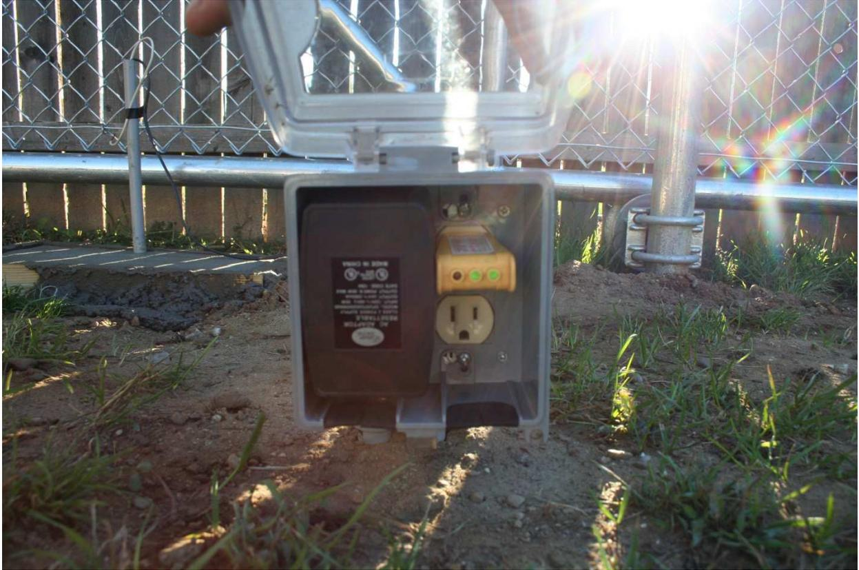
This is the modified outlet box in the yard. I removed the left outlet and wedged the 24 VAC transformer in place. On the right is a circuit tester that confirms that all the wiring is correct. The whole thing is in a weather-resistant case. You can find this at Lowes easily.
