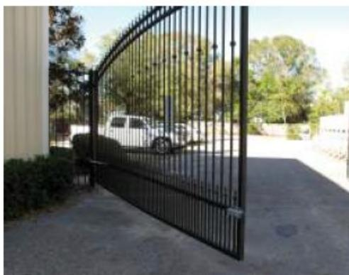
Manually unlock the gate, then move it half-way and re-engage. Activate using Push 1 button (as shown above) The gate should run open. Press Push 1 again and it should run closed. The gate is now set up for regular usage.
